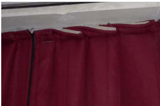
Photos of assembly of test specimen
